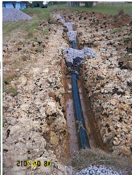
Perforated pipe covered in stone with straw separation layers
