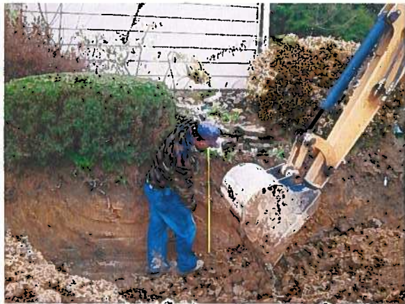
Excavate a drywell at least 10' from foundation
