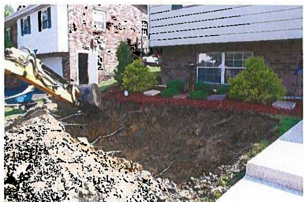
Excavate rain garden at least 10' from foundation
