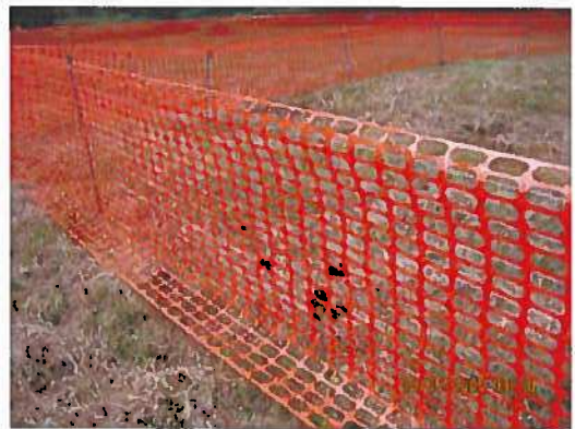
Fencing protects areas from compaction
