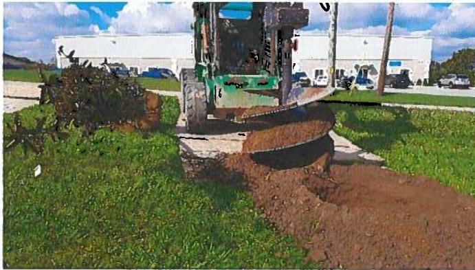
Plywood sheets protect lawn from compaction
