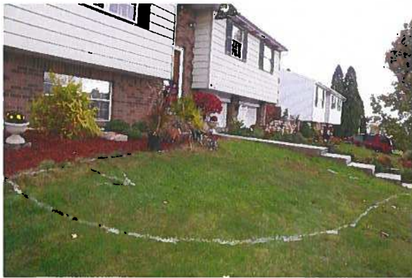
Mark rain garden location to avoid utilities
