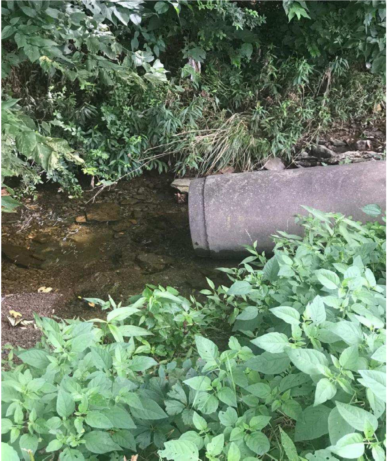
Outfall #17 of UNT #1 to the Monongahela River along Grand Boulevard
