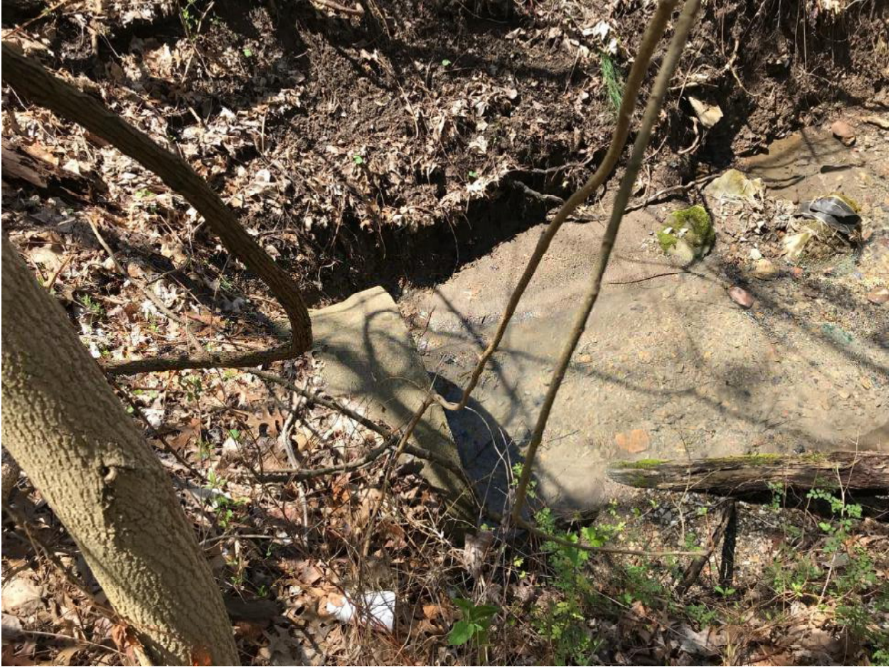
Outfall #3 of UNT #2 to the Monongahela River along Tyrol Boulevard
