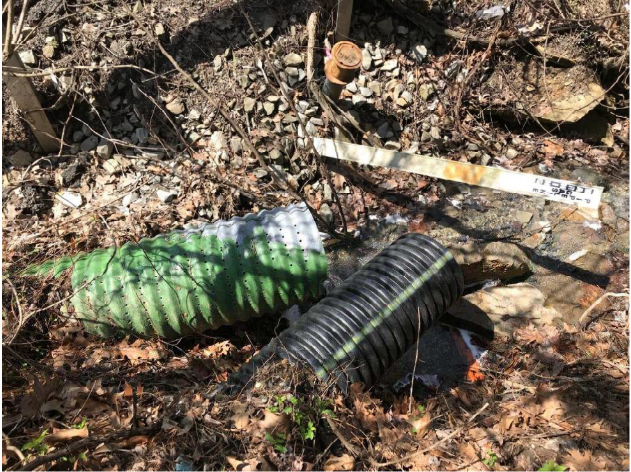
Outfall #2 of UNT #2 to the Monongahela River along Tyrol Boulevard
