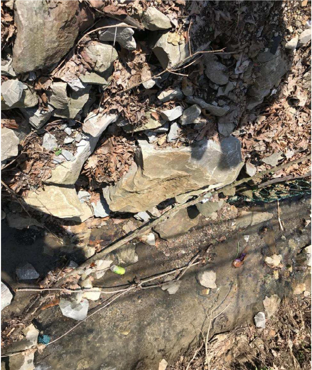
Outfall #6 of UNT #2 to the Monongahela River along Tyrol Boulevard
