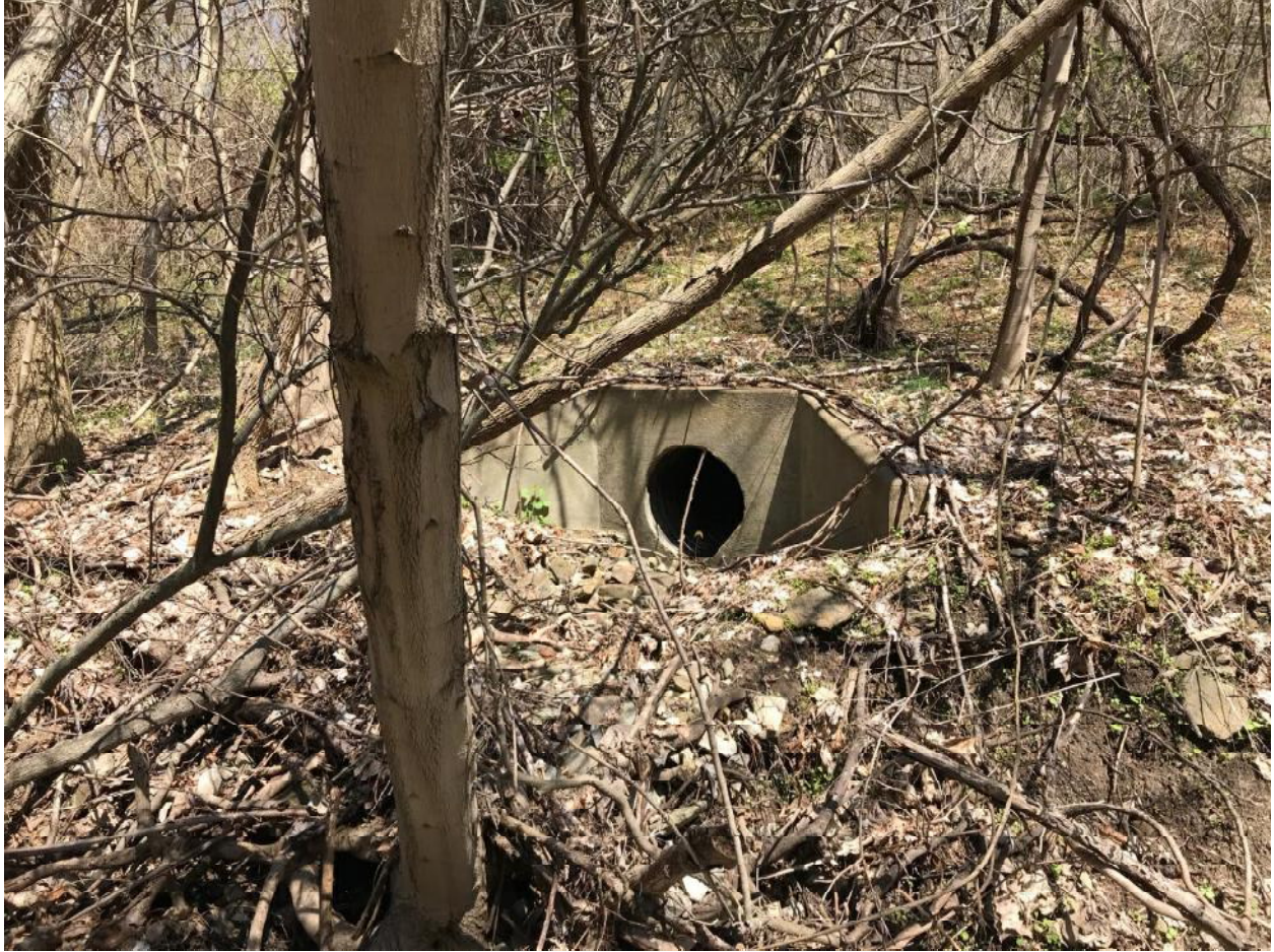
Outfall #5 of UNT #2 to the Monongahela River along Tyrol Boulevard
