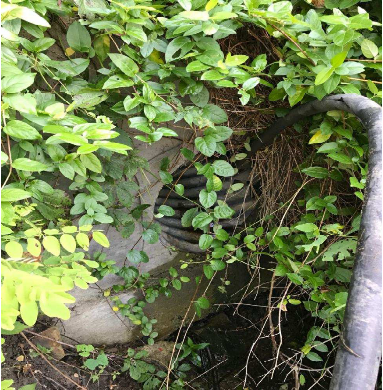
Outfall #18 of UNT #1 to the Monongahela River along Grand Boulevard
