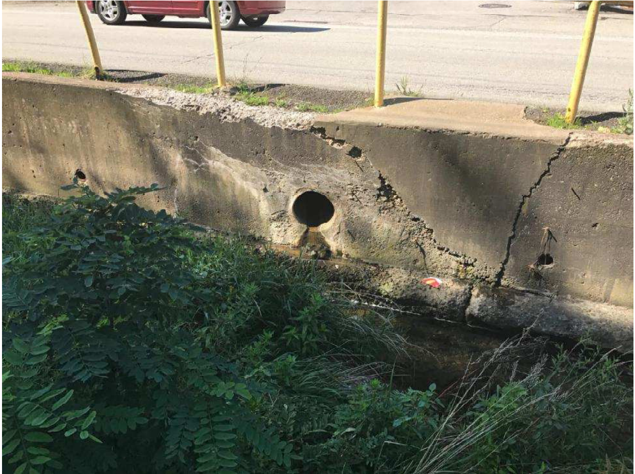
Outfall #19 of UNT #1 to the Monongahela River along Grand Boulevard
