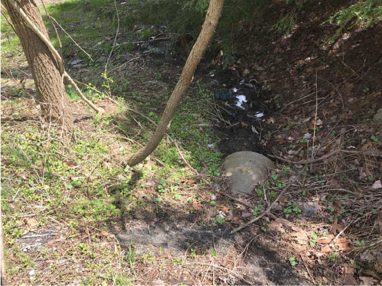
Outfall #3 of UNT to Speers Run along State Road
