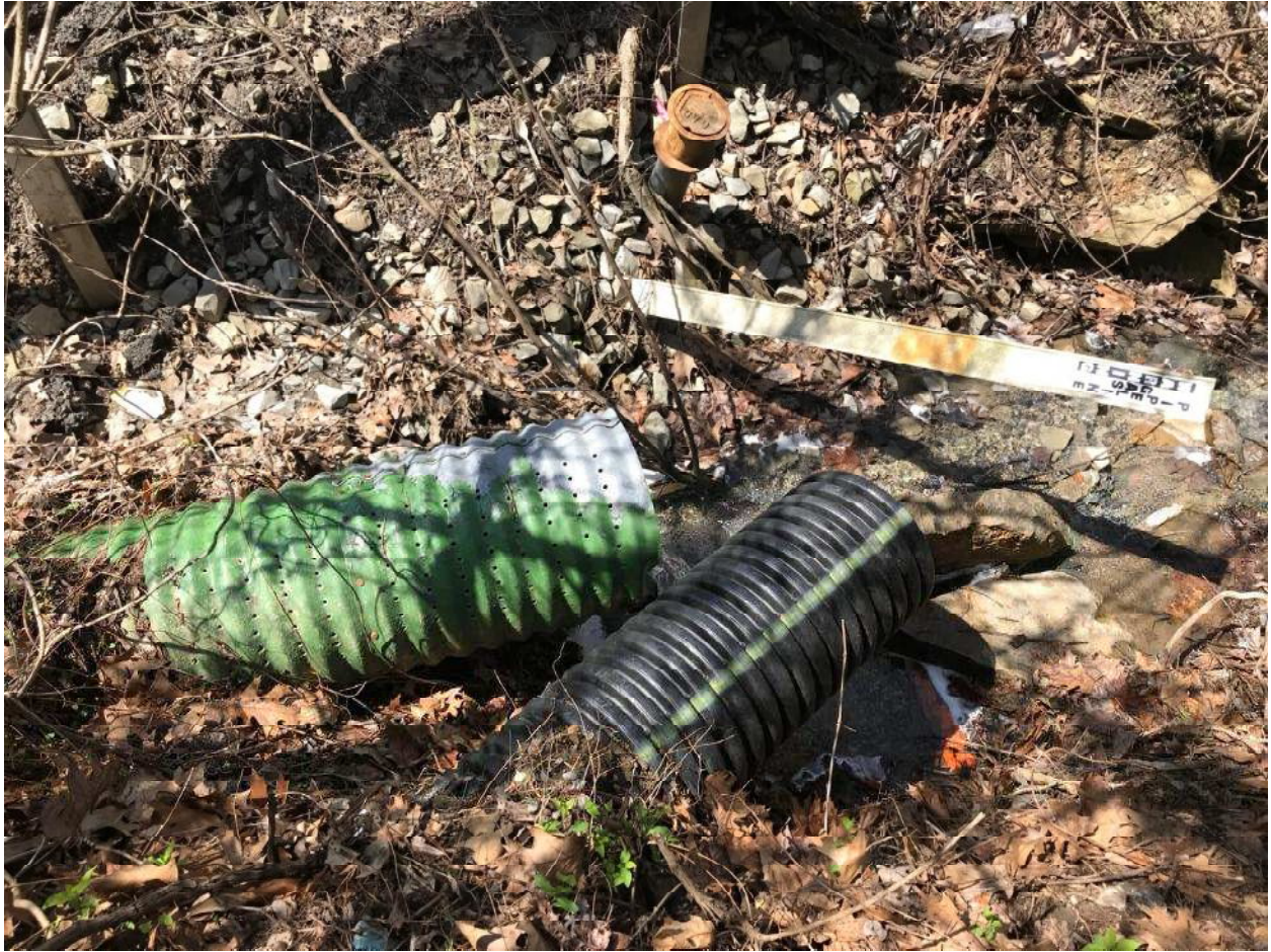
Outfall #1 of UNT #2 to the Monongahela River along Tyrol Boulevard
