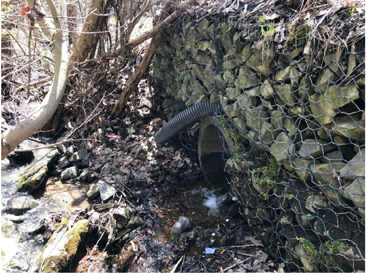
Outfall #4 of UNT #2 to the Monongahela River along Tyrol Boulevard
