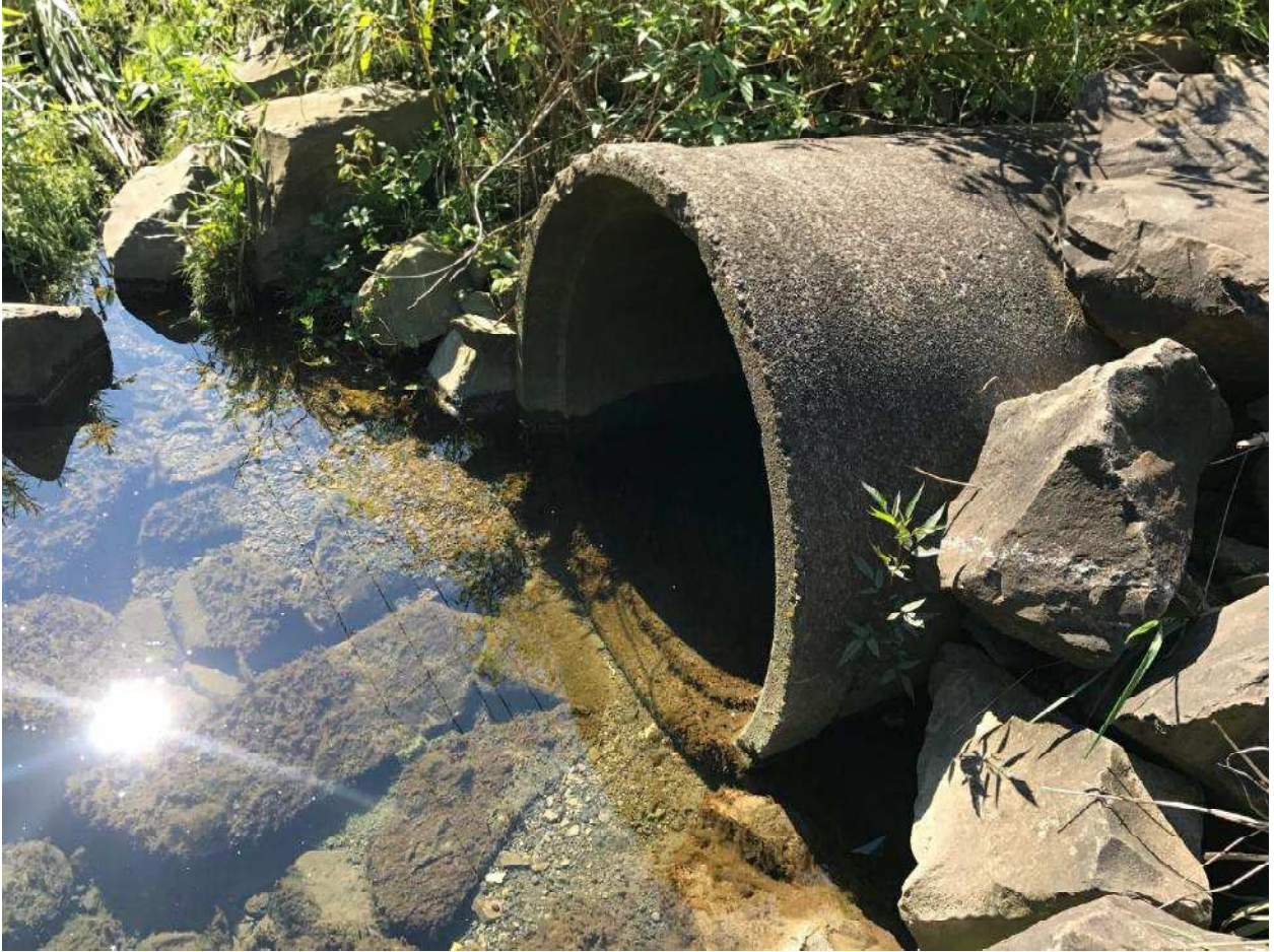
Outfall #16 of UNT #1 to the Monongahela River along Grand Boulevard
