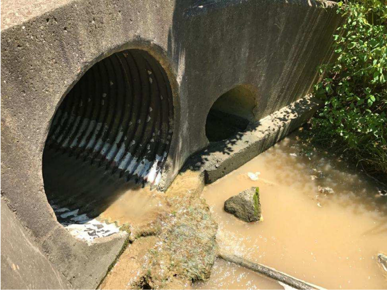
Outfall #7 of UNT #1 to the Monongahela River along Grand Boulevard
