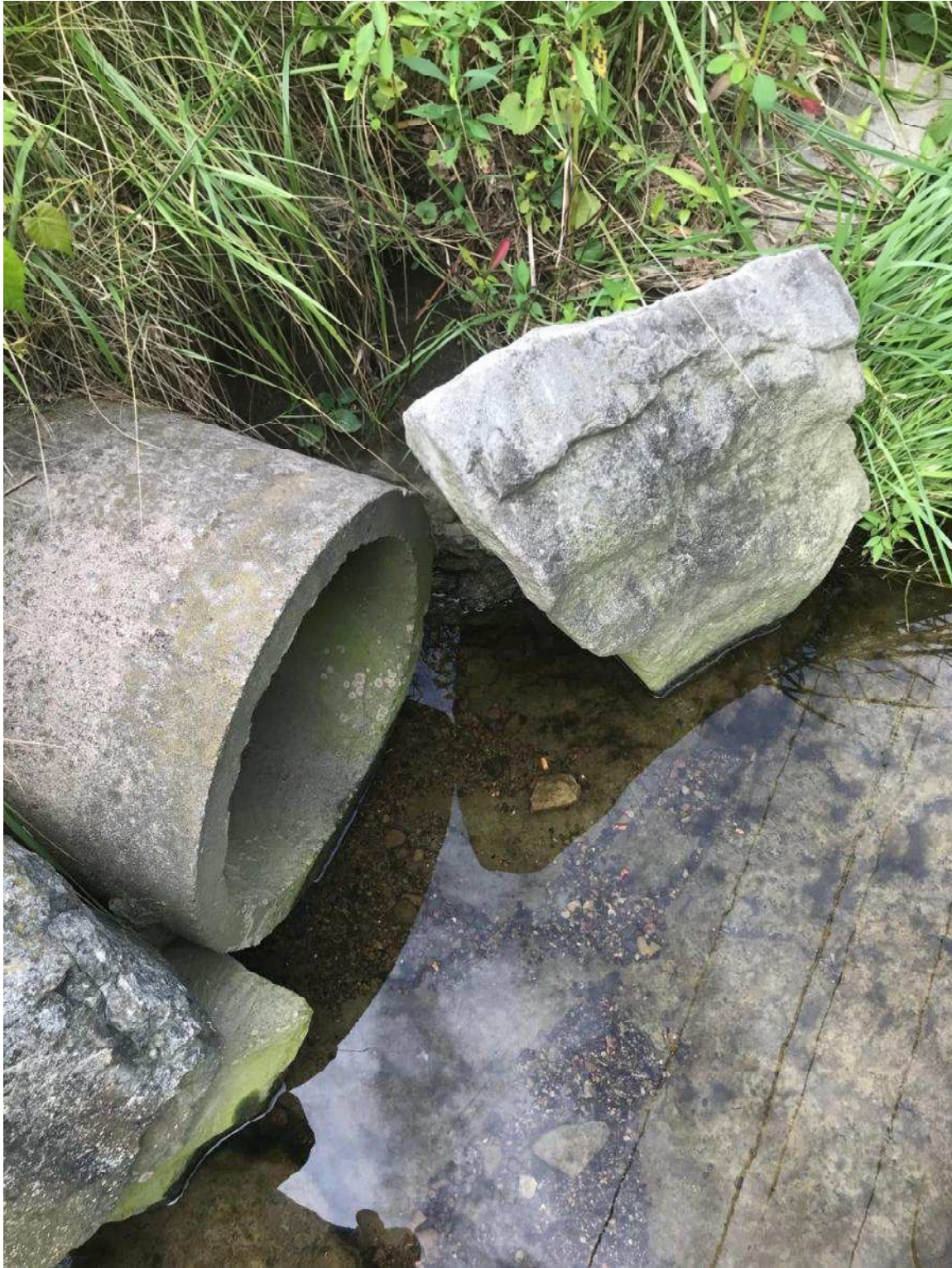
Outfall #15 of UNT #1 to the Monongahela River along Grand Boulevard
