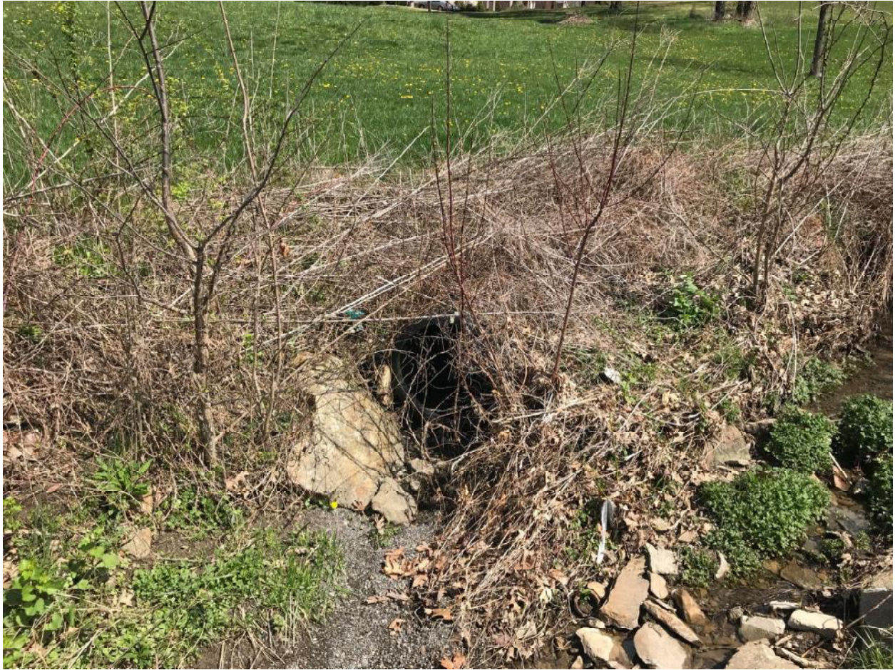
Outfall #12 of UNT #1 to the Monongahela River along Grand Boulevard
