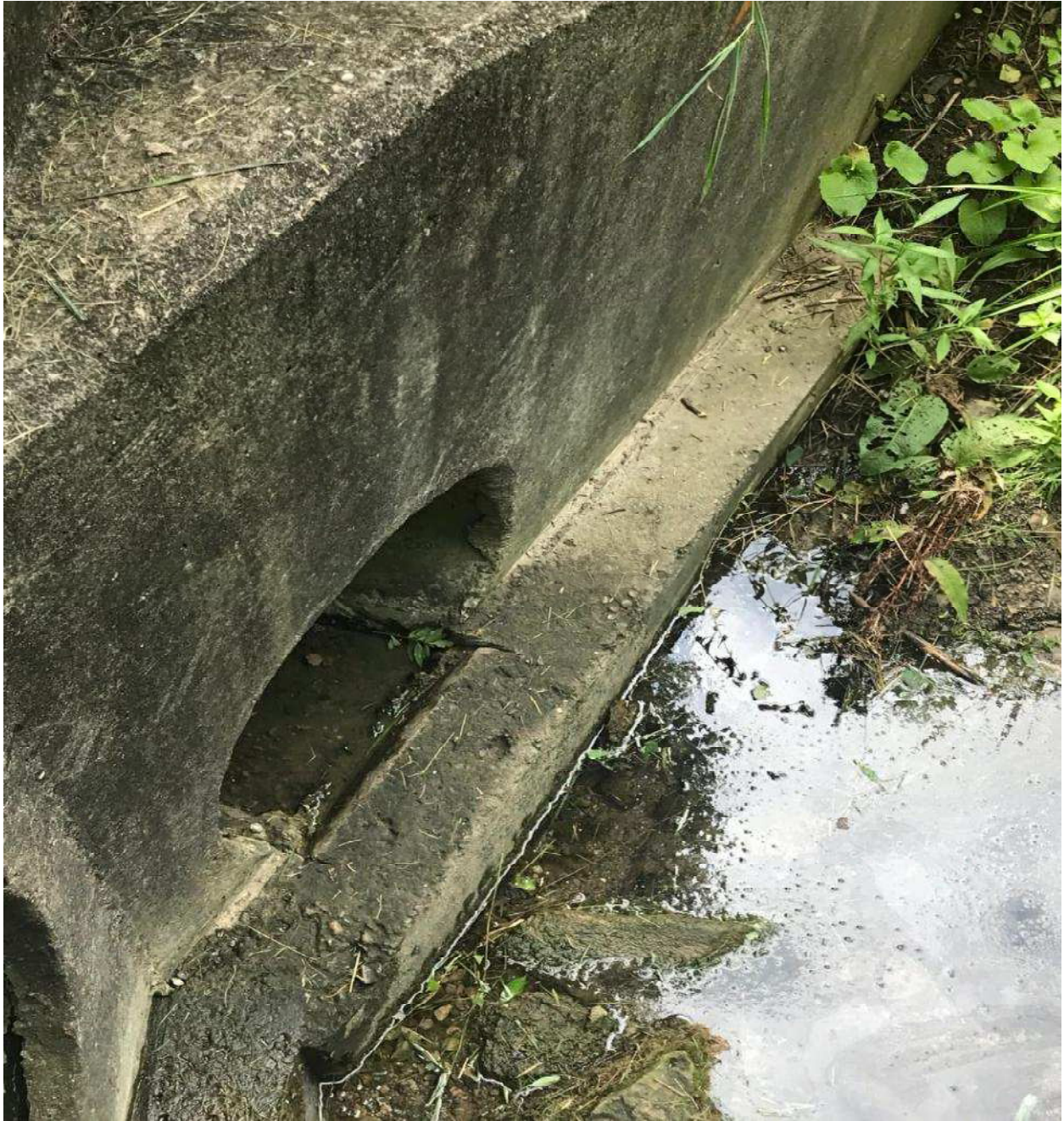
Outfall #8 of UNT #1 to the Monongahela River along Grand Boulevard
