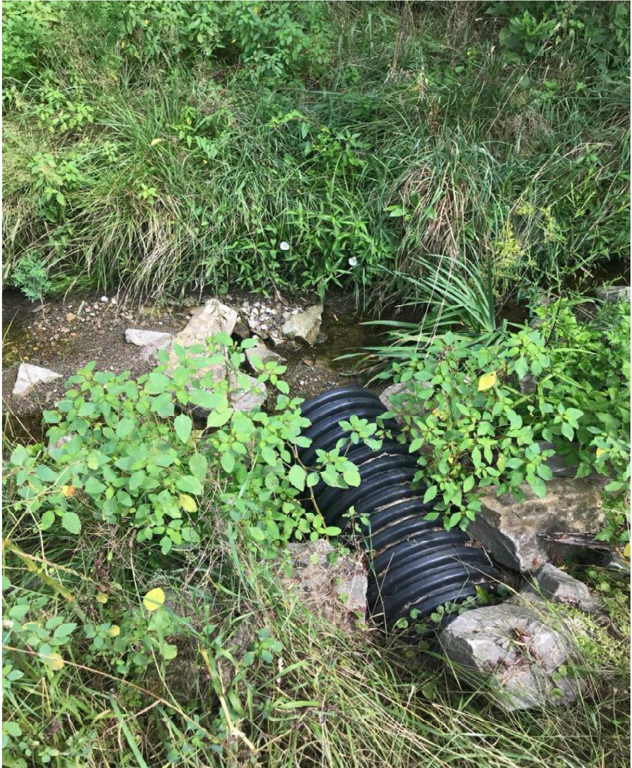
Outfall #10 of UNT #1 to the Monongahela River along Grand Boulevard
