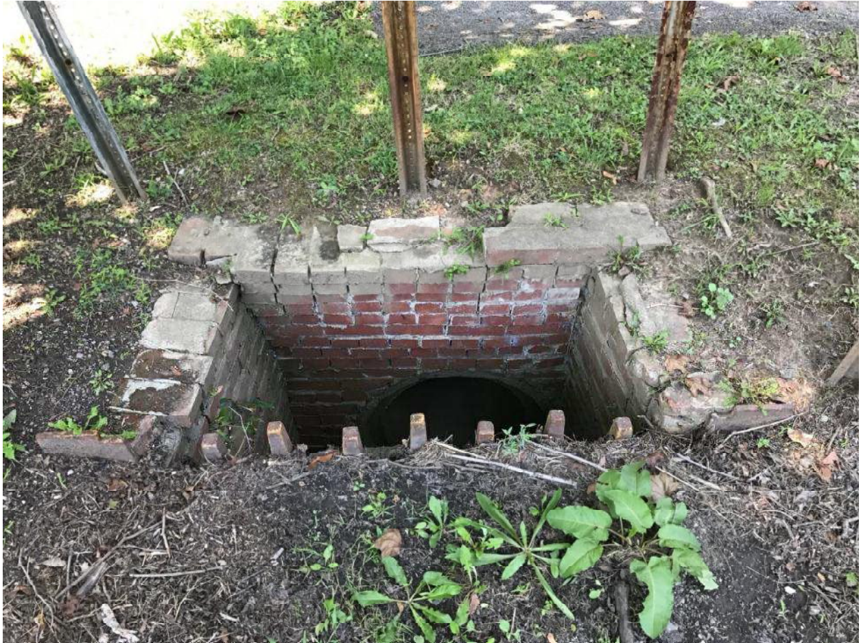
Outfall #6 of UNT #1 to the Monongahela River along Grand Boulevard
