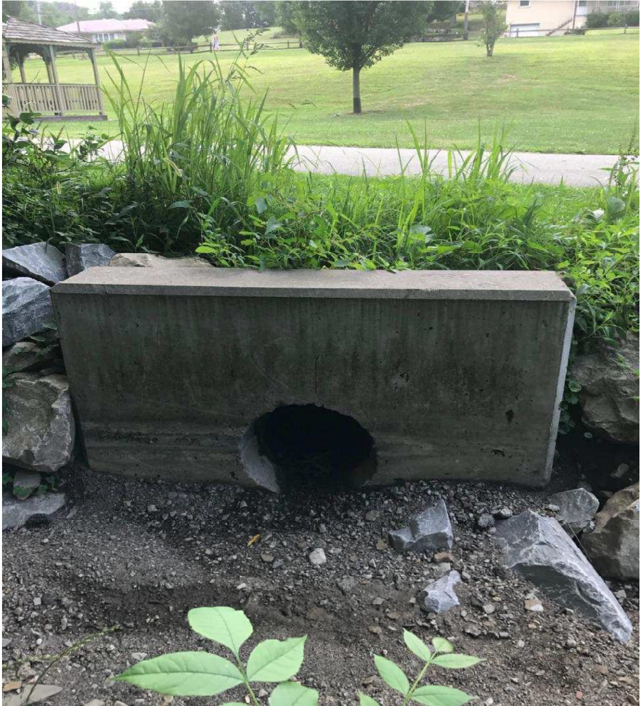
Outfall #11 of UNT #1 to the Monongahela River along Grand Boulevard
