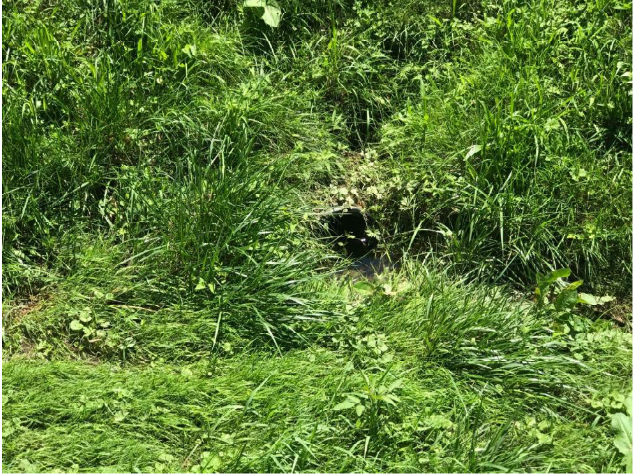
Outfall #5 of UNT #1 to the Monongahela River along Grand Boulevard
