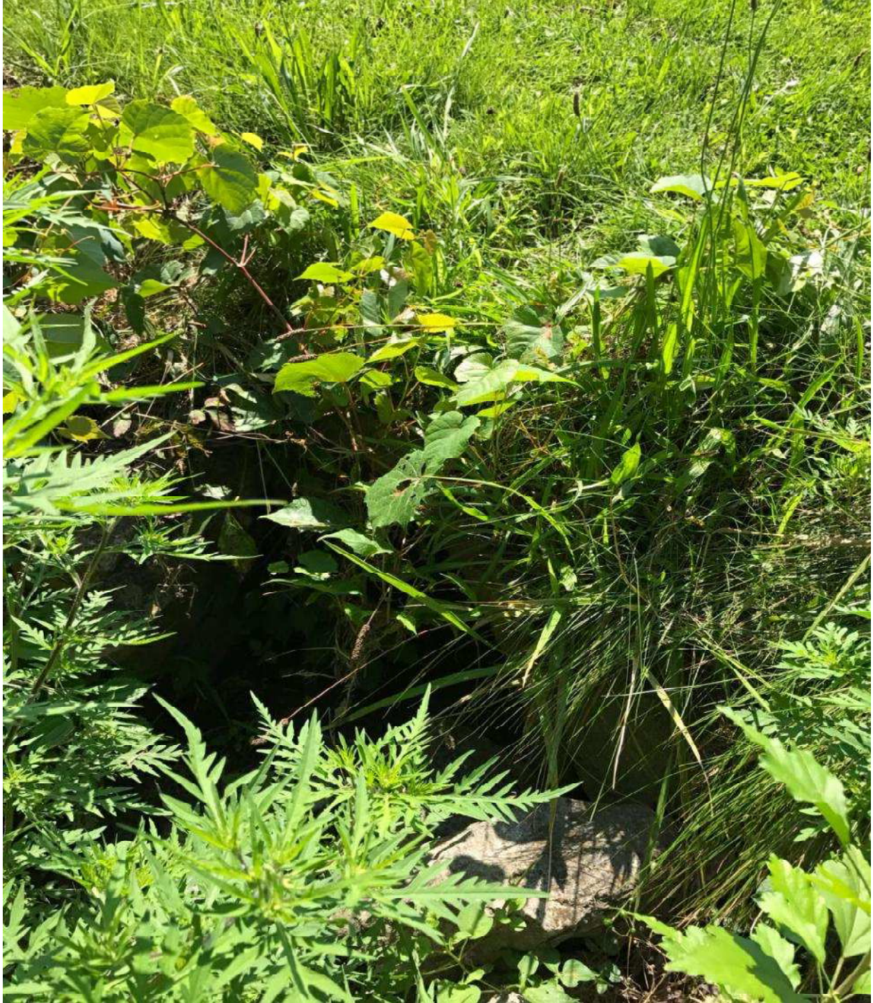
Outfall #9 of UNT #1 to the Monongahela River along Grand Boulevard 15" CPP (View of obscured by heavy vegetation)
