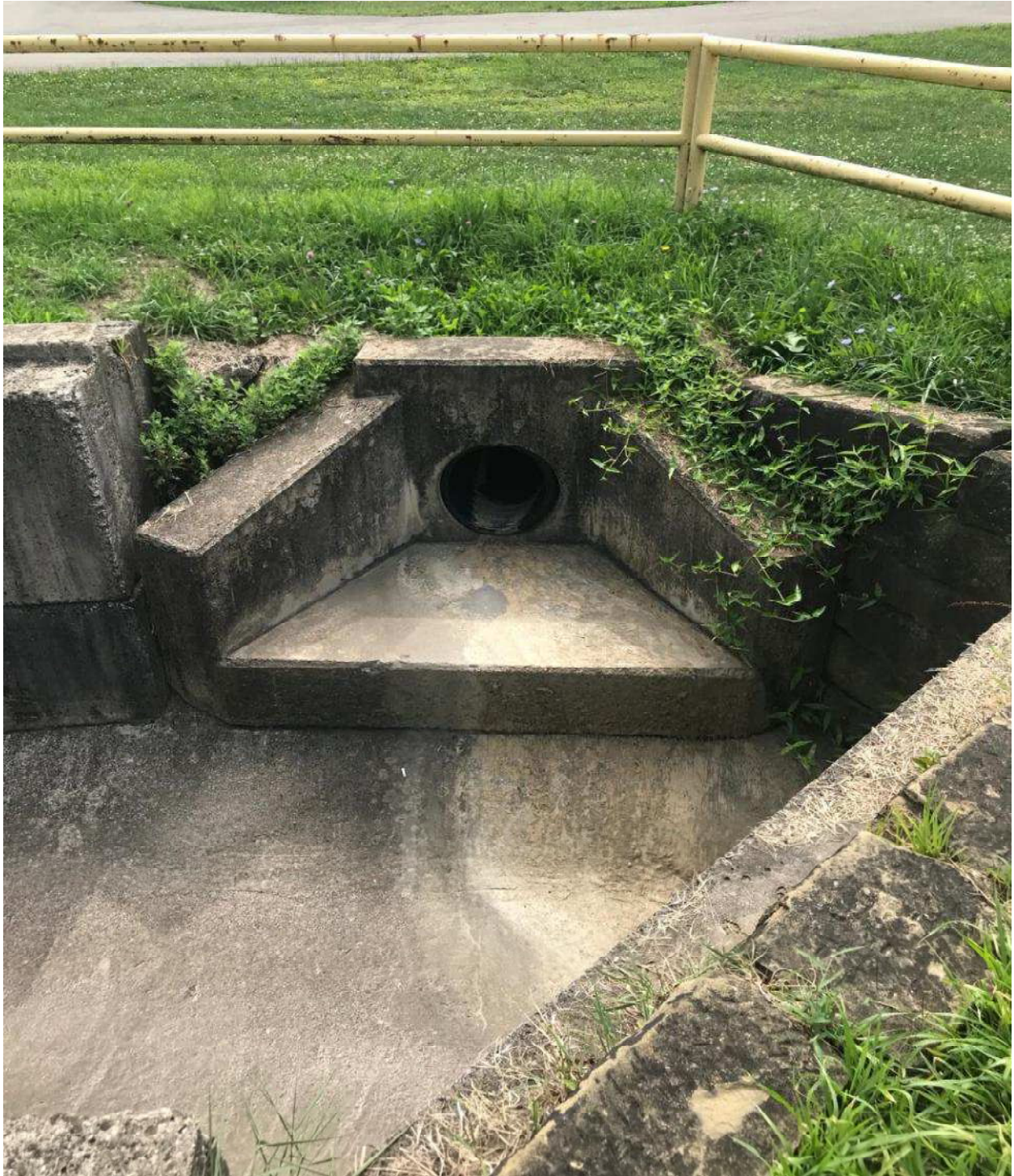
Outfall #14 of UNT #1 to the Monongahela River along Grand Boulevard
