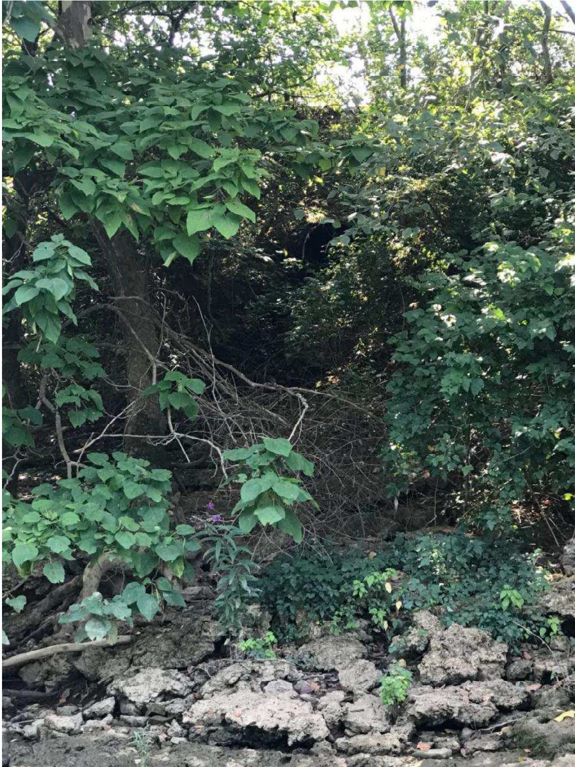
Outfall #SS005 of the Monongahela River. Outfall obscured by heavy vegetation.
