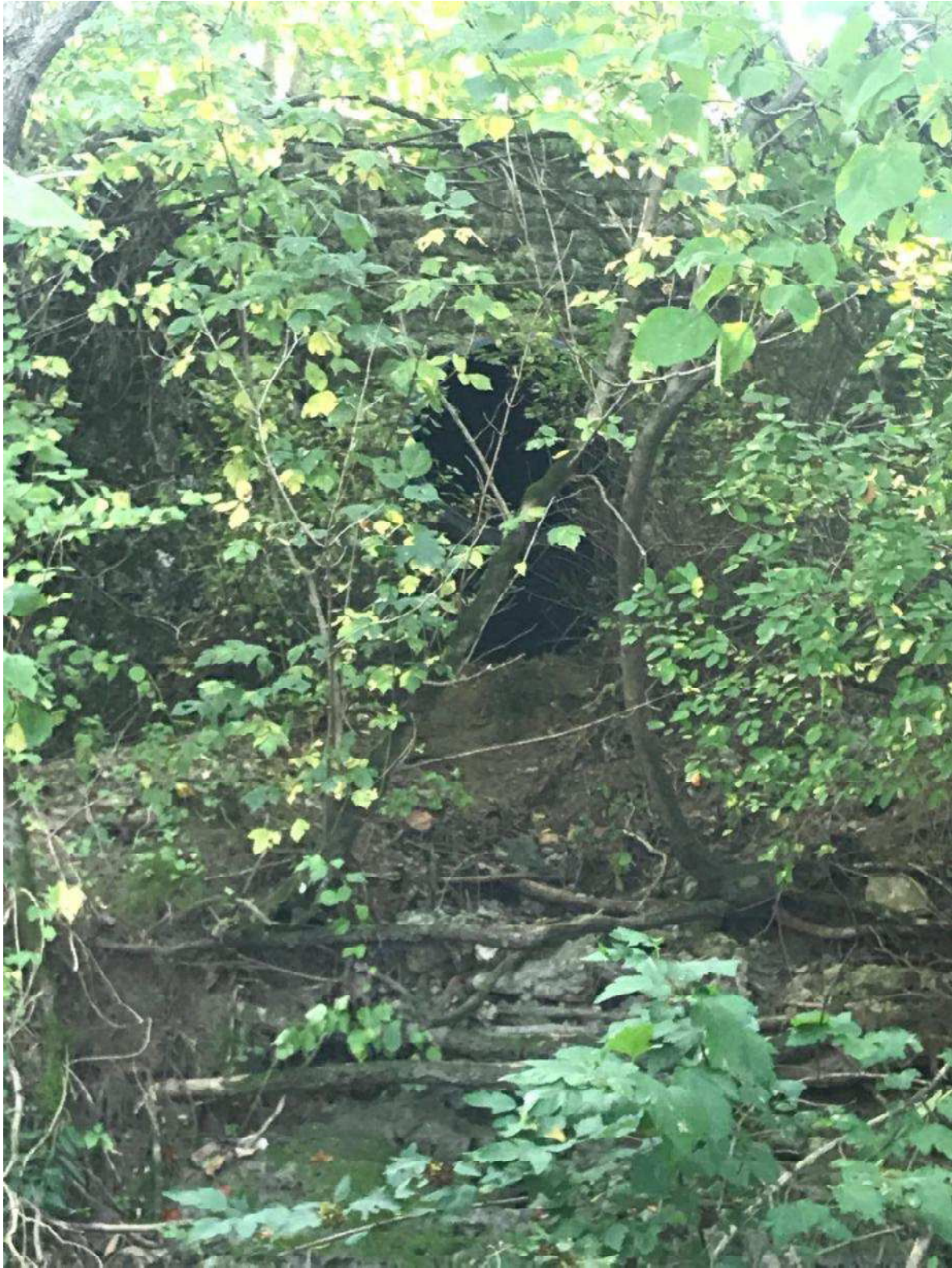
Outfall #SS003 of the Monongahela River. Outfall obscured by heavy vegetation.
