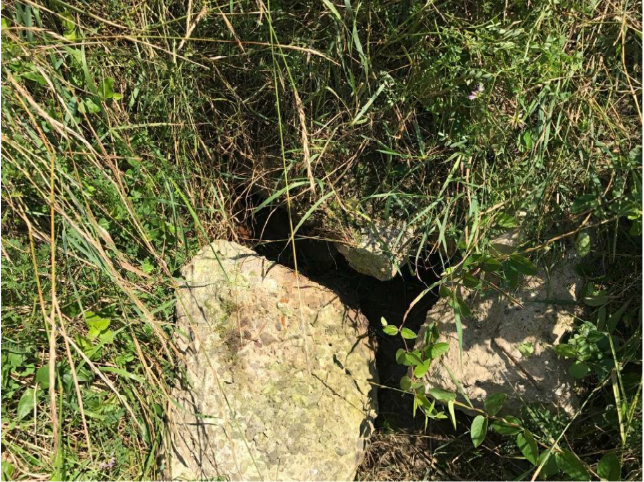
Outfall #2 of UNT #1 to the Monongahela River along Grand Boulevard
