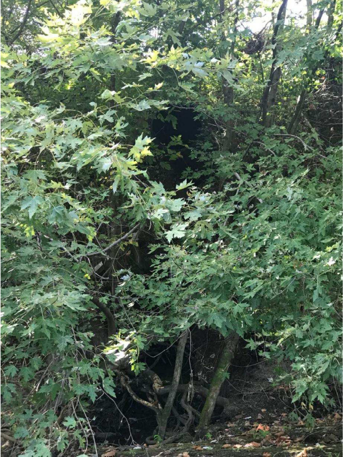
Outfall #SS006 of the Monongahela River. Outfall obscured by heavy vegetation.
