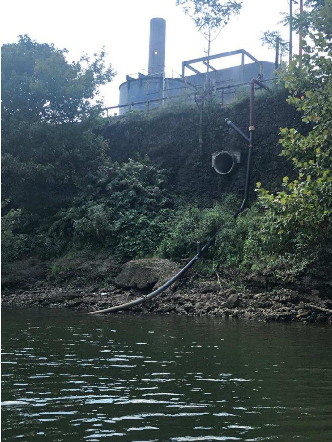
New Outfall D of the Monongahela River. Pipe outlet coming from Mill property above.
