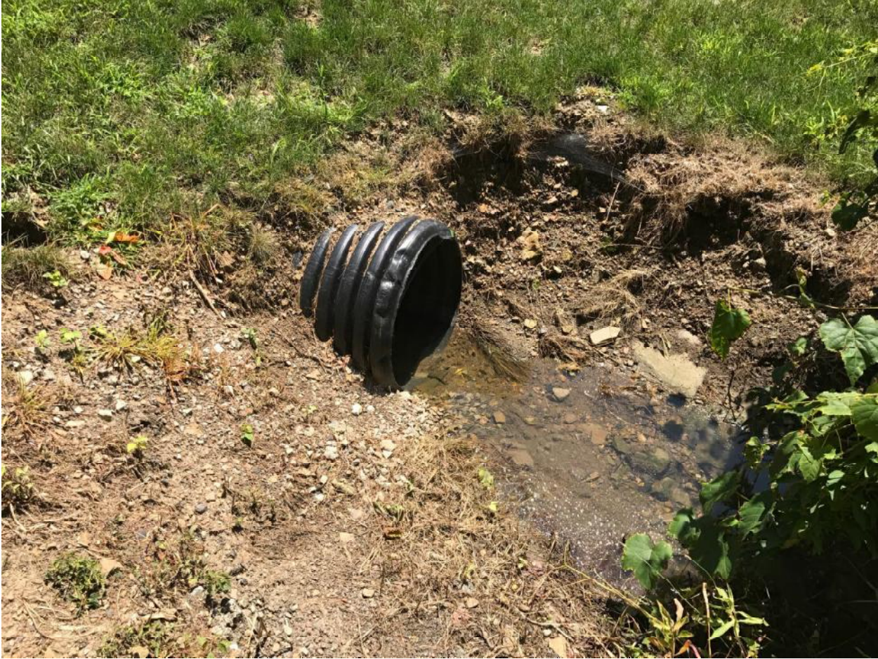
Outfall #4 of UNT #1 to the Monongahela River along Grand Boulevard
