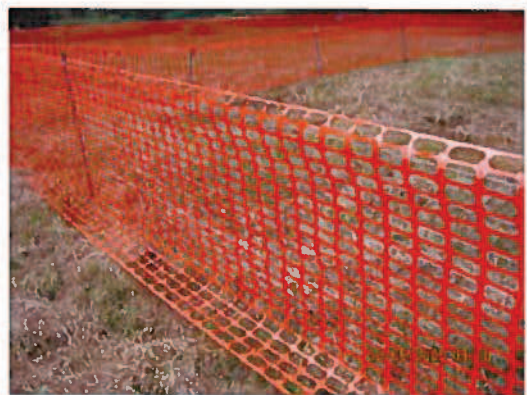
Fencing protects areas from compaction
