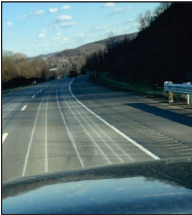
Figure 11: An example of anti-icing BMP, where a brine solution is placed on a roadway prior to a winter storm. Photo credit: Darrel Lewis, Armstrong County.
