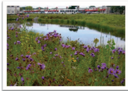
Wet ponds are relatively easy to construct and maintain. Their stormwater management functions include peak rate control and water quality improvement. Photo: rwmwd.org
