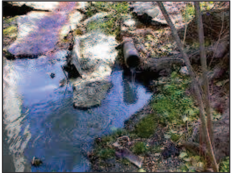
Figure 5: Illicit discharge (Source: EPA IDDE Manual: https://www3.epa.gov/npdes/pubs/idde_manualwithappendices.pdf )
