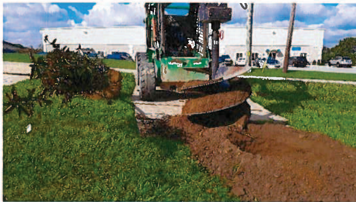
Plywood sheets protect lawn from compaction
