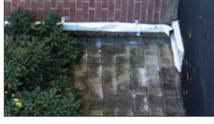
Downspouts for roof runoff
