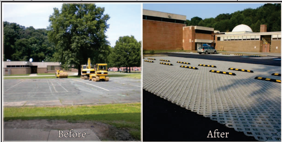
New parking at Valley High School with permeable pavers. Photos: Westmoreland Conservation District
