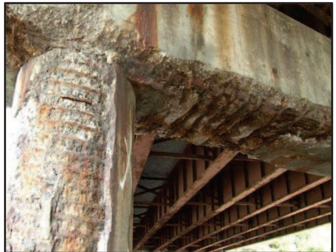
Figure 4: Significant damage from many years of salt and deicing chemical use from a leaking expansion joint. Source: Bridge retrofit using fiber reinforced polymer, cenews.com
