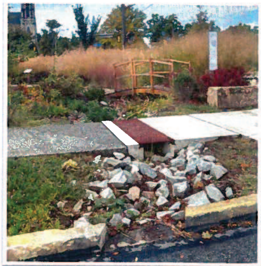
Bioswales (above) are a structural BMP that can help mitigate the effects of stormwater once a site has been developed.
