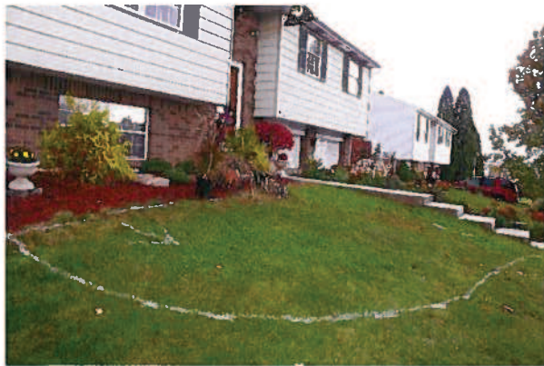
Mark rain garden location to avoid utilities
