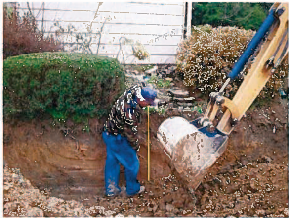
Excavate a drywell at least 10' from foundation
