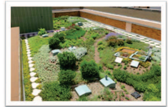
A green roof was installed on the Allegheny County Office Building (above) in 2010 as a demonstration project. There are four types of green roof technologies and extensive monitoring equipment in place. Photo: eislerlandscapes.com
