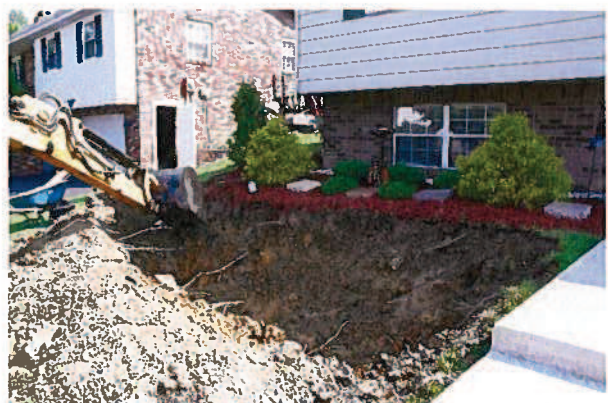
Excavate rain garden at least 10' from foundation
