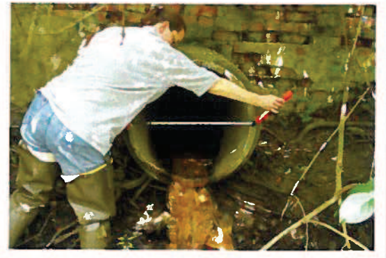
MCM #3 under the MS4 program requires regular screening of stormwater outfalls to detect any illicit discharges. Photo: water.epa.gov
